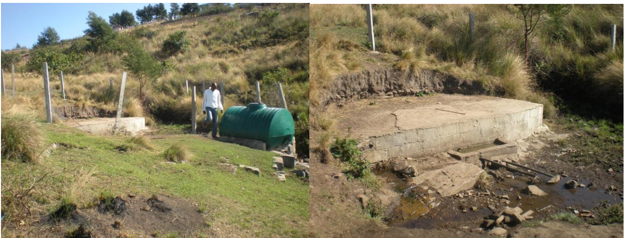
Figure 4.10: Borehole used for water supply (tank supplied by ORTDM)
